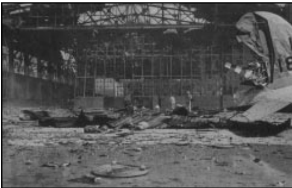
The effects of a good strafe – note the damage to this hangar – are comparable to bomb damage.
